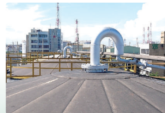
Breather valve connecting pipe setup
