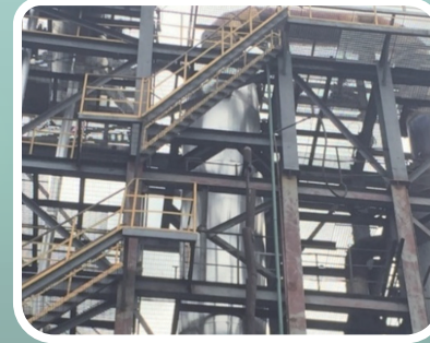
Online heat recovery boiler (overall heat exchanger section) of Maanshan Plant, Greater China
