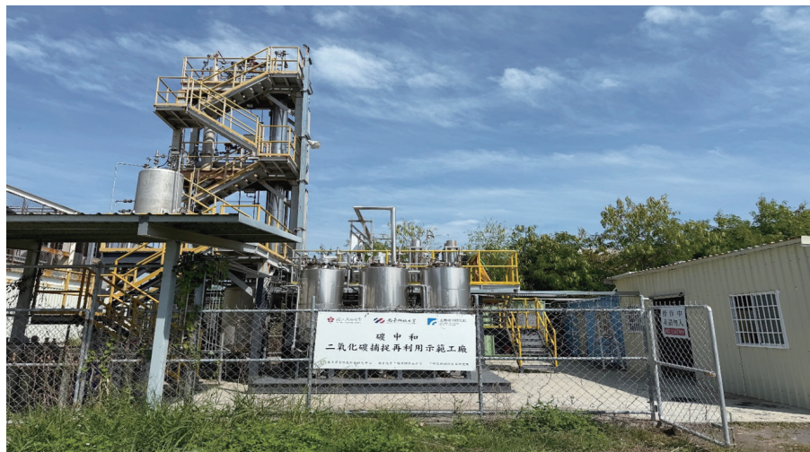
The project utilizes Professor Chen's patented potassium acetate sorbent to replace traditional amine-based absorbents, achieving low-energy desorption of CO 2 . Additionally, it incorporates a microbubble CO 2 capture device co-developed with Professor Chen's team to enhance capture efficiency. The goal is to develop sustainable technology with commercial value.
