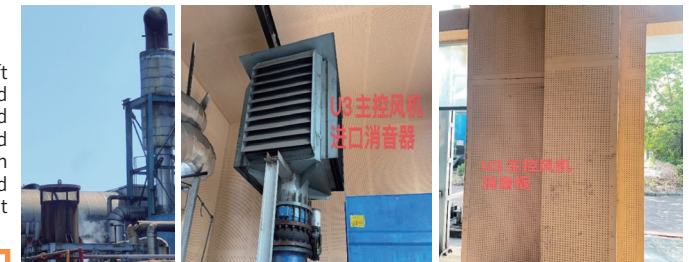
Inlet Silencer for U3 Main Control Fan
