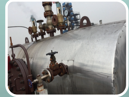
Online heat recovery boiler (steam drum) of Maanshan Plant, Greater China
