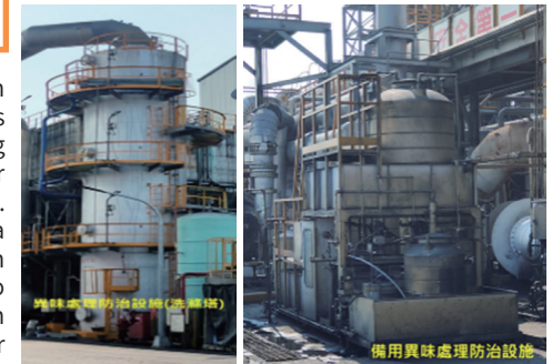
Odor treatment and control facilities (scrubbing tower)
