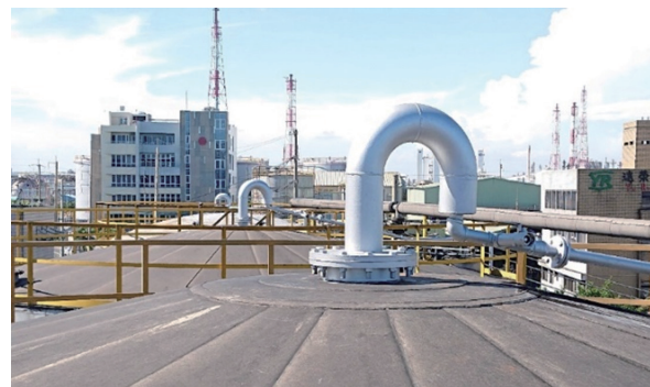
Breather valve connecting pipe setup
